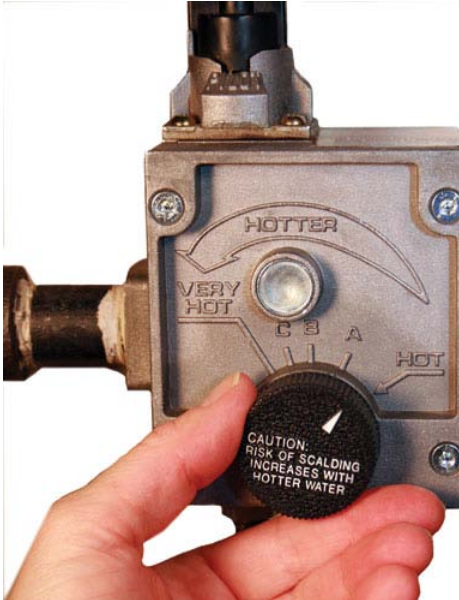
Photo: A thermostatically controlled gas valve.
